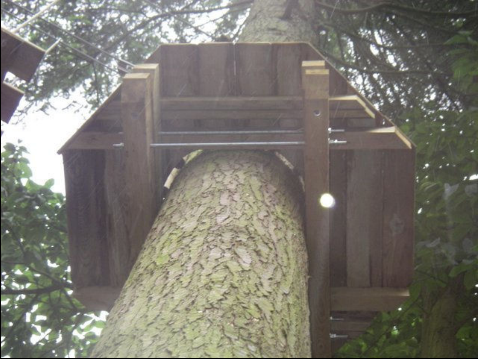
Example of Brace and Platform Construction
